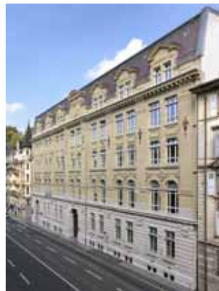
THE BUILDING AT 19 RUE DU DR CÉSAR-ROUX IN LAUSANNE, renovated to welcome the Santé Vaud School of Advanced Studies (HESAV). © Lionel Henriod
